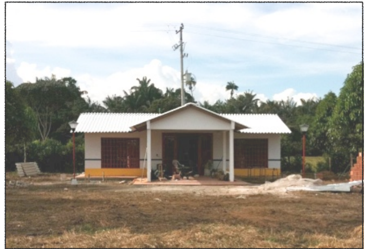
The first cabin has been completed.
